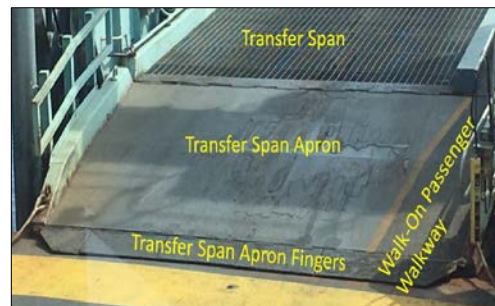
Figure 7 Transfer span components
